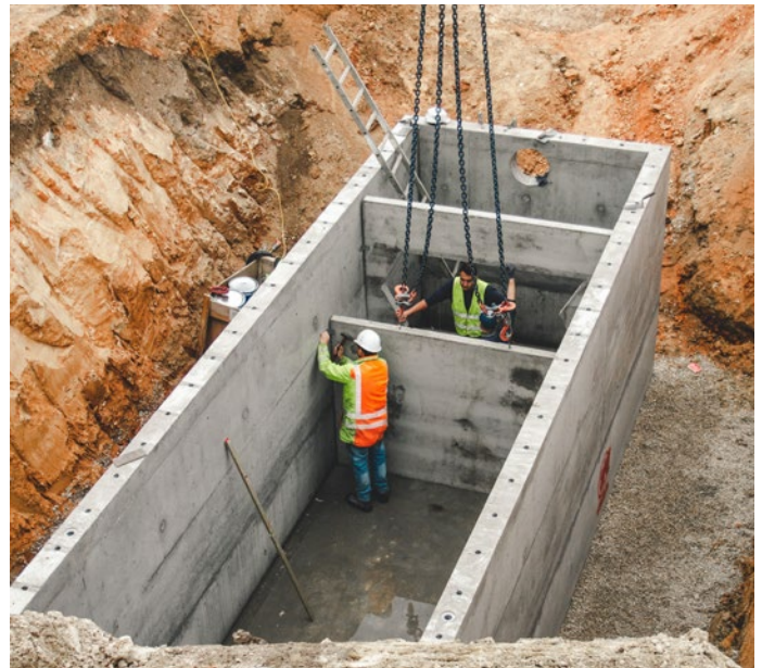
Buried under the site of the Föhrenberg service station on the A2 in the direction of Graz is a gigantic shaft structure that was produced jointly by the Kirchdorfer Concrete Solution family as a special precast element.
