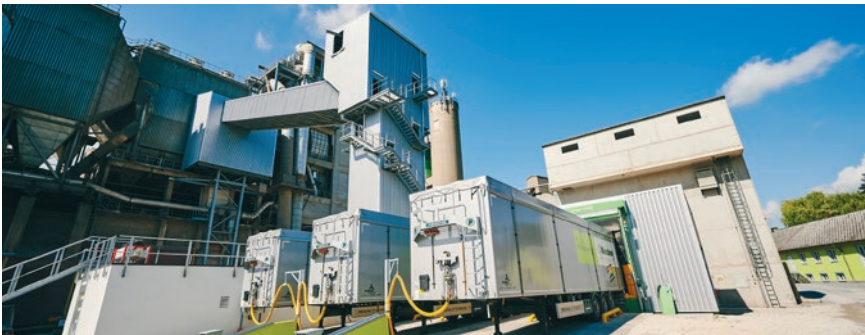
New logistics concept for the delivery of substitute fuels: An intermediate storage facility for the new terminals was built at the rear of the plant. On this occasion, the entire traffic flow into and out of the plant is also being reorganized.
