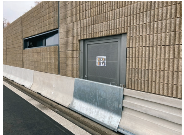
Barrier-free escape door, integrated radar unit: The new PHONOBLOC® DB NBF noise barriers on the A81 in the Zuffenhausen area leave nothing to be desired.
