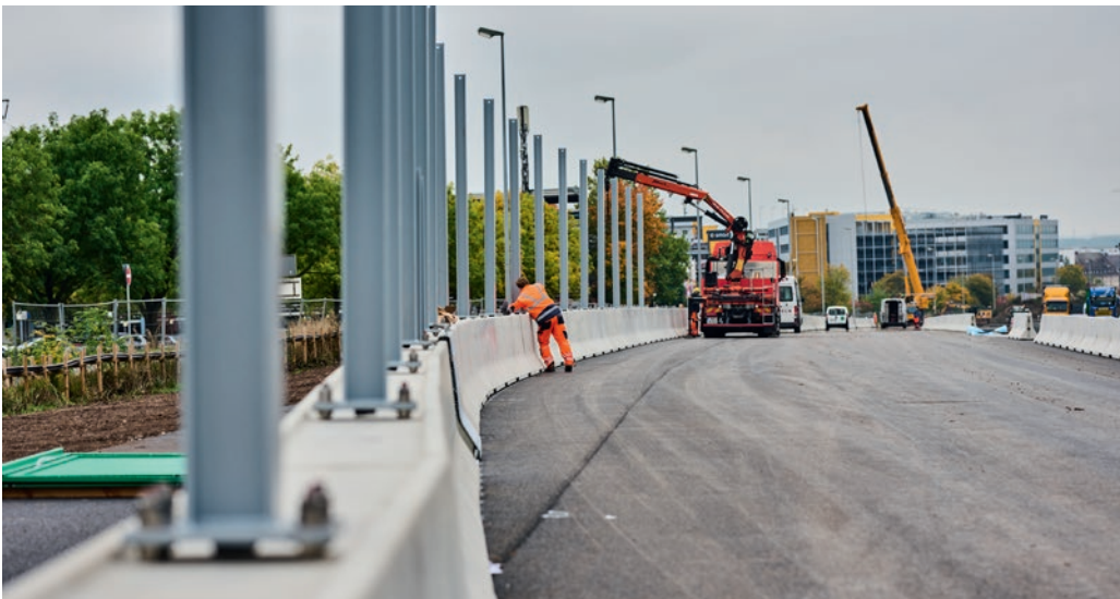
"All-round carefree package": Installation of noise protection and restraint systems on the A81/Sindelfingen.
